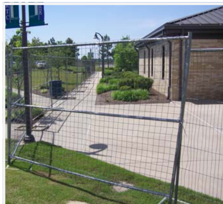
Buildings on the west side of the BRTC campus remain fenced off while work is in progress.
