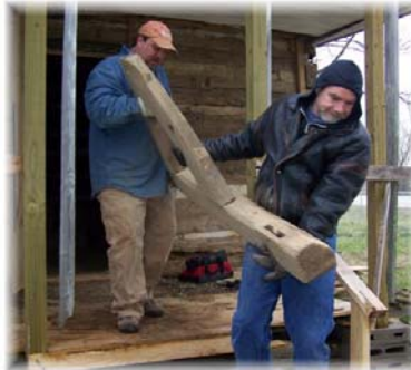
Jared Evans and Randy Tipton of Fayetteville carry part of the loom out of the Rice House for safekeeping during the restoration of the house itself. The loom has been donated to BRTC for restoration.
